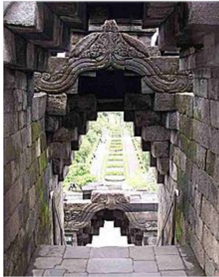
Stone corbelled arches at Borobudur in Java, Indonesia. Note the "T"-shaped central stones.
